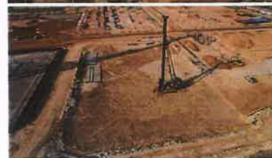
Retention Pond Pilot Pile driven
