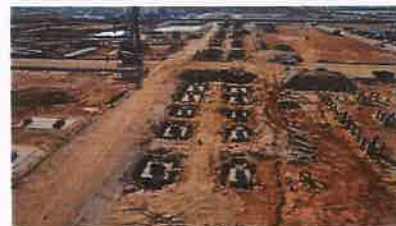
Pipe rack Foundation
